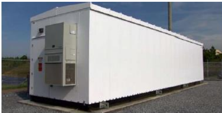
Figure 6 Typical 40 ft modified shipping container for battery energy storage (extracted from Edify Memo)
